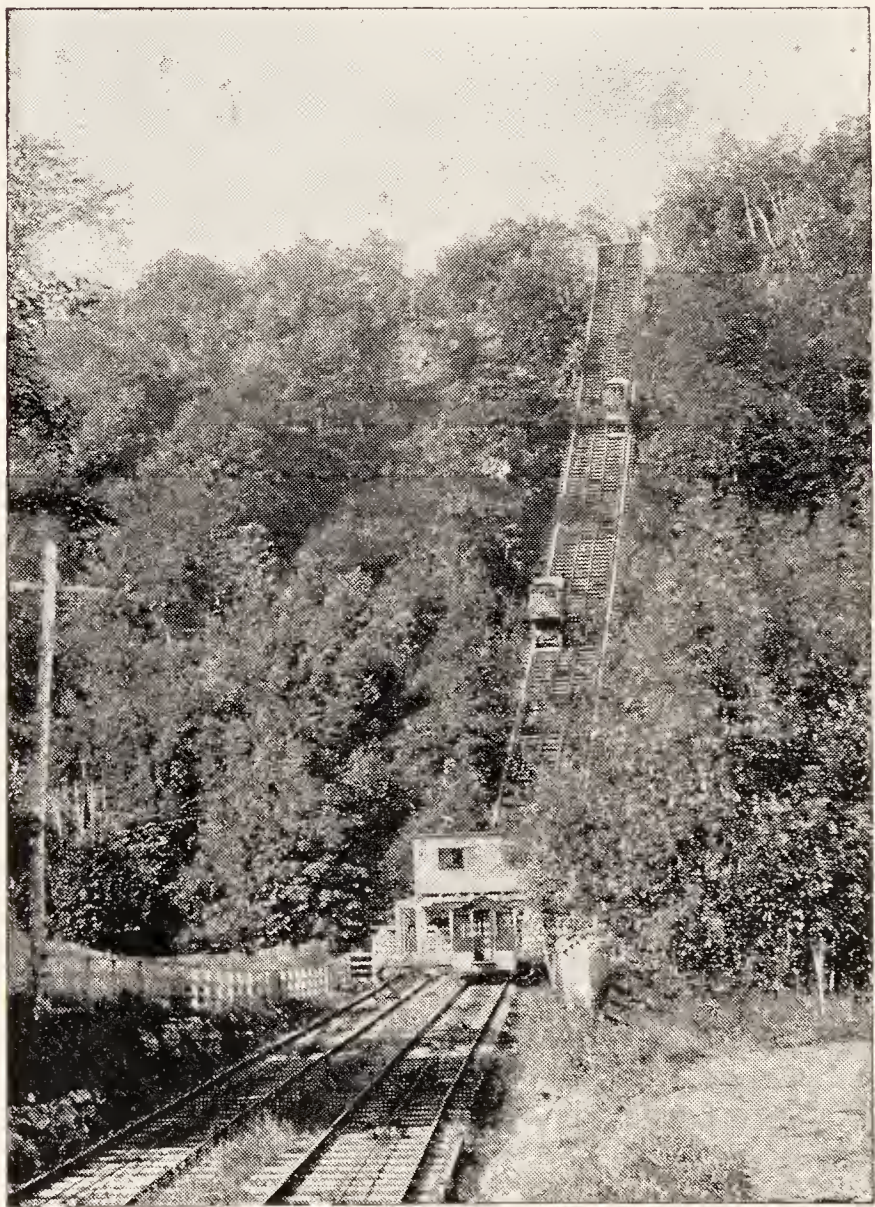
ELEVATOR ON THE EASTERN SLOPE OF MOUNT ROYAL.
